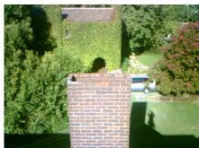
The chimney crown is deteriorated and needs to be repaired to prevent further
