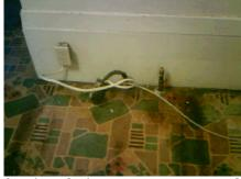
Gas line is not capped, electric outlet is not secure or protected by conduit. A licensed contractor, experienced in this field, should further evaluate this condition. Bootleg 110 volt circuit has been taken from 220 volt outlet. 110 volt outlet is not properly protected by circuit breaker. *THIS IS A HEALTH/SAFETY CONCERN*.
