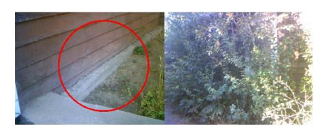
Vegetation limits access to the exterior surfaces. Earth to wood clearance is: Poor at: all areas where concrete is poured over wood members.
