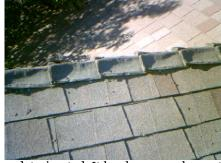
Pieces of the ridgecap are deteriorated, It has been my observation the high profile ridge cap that has been installed deteriorates at a rate faster than the field materials. Depending on conditions, the ridge might need to replaced after 10-15 years. Repair/replace as needed.
