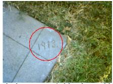
Concrete. There are cracks that appear typical for a house of this age. We recommend sealing any cracks in the walkway slabs to prevent further water intrusion. Installed in 1913.
