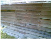
All horizontal trim should be regularly maintained to prevent water infiltration and material deterioration. This usually includes caulking and painting. Paint is no longer providing the protection needed.
