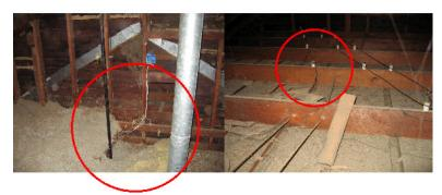
I observed splicing of modern wiring to the old knob & tube that does not conform with modern splicing guidelines = Recommend further evaluation/repair by a licensed Electrician. Noted line splices in the attic without the use of proper J-boxes and covers = Repair. Knob & Tube wiring is covered with insulation = This may present a Fire hazard. A licensed contractor, experienced in this field, should further evaluate this condition.
