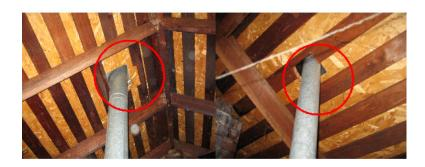
Clearance to combustable materials does not meet manufactures recommendations. 6" clearance to single wall and 2" clearance to double wall is common. Both the furnace and water heater.
