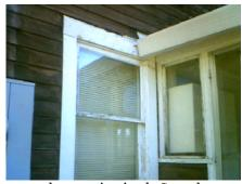
Windows are old and have not been maintained. Some have material deterioration.
